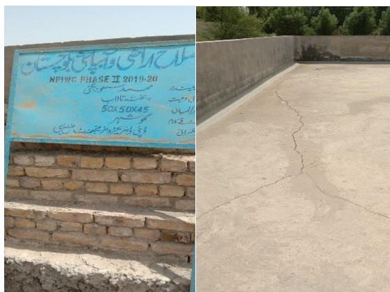
Cracks in Bed of Water Storage Tank - Saud Bugti
