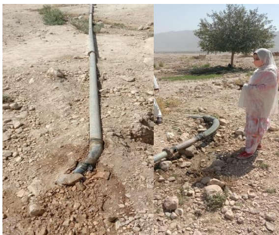
View of PVC Watercourse – Leakage of Water at Joint
