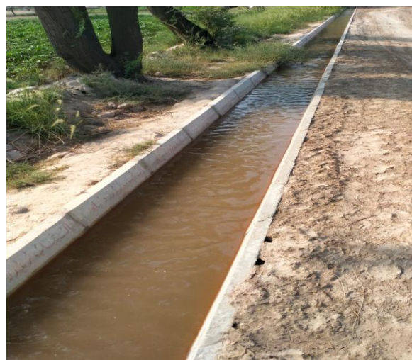
Holes show Improper Compaction of Backfilling
