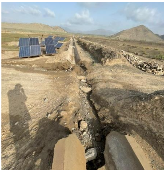
Picture showing Damaged Watercourse
