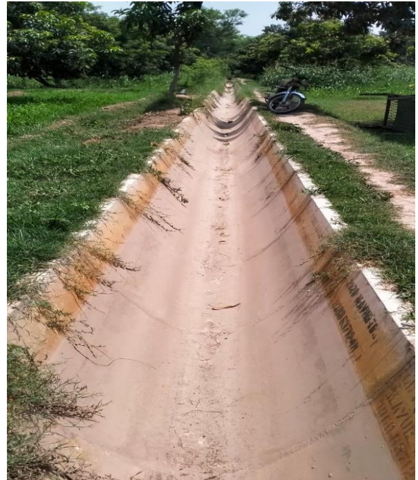
View of Parabolic W/C – Needs removal of Weeds
