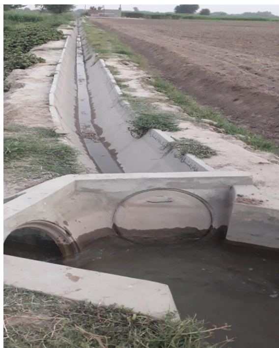
Controlled Structure of Parabolic Watercourse
